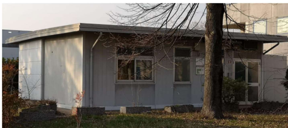
Figure 21. Demonstration site No 1 in Padova, Italy
