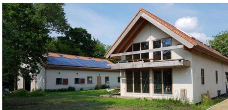
Figure 20. Demonstration site No 3 in Putte, Belgium
