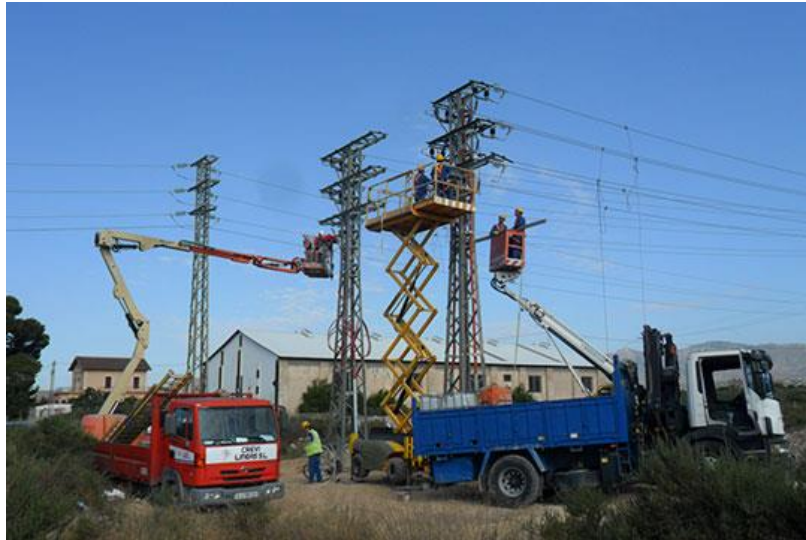
Figure 34 Maintenance works on a distribution power line.
