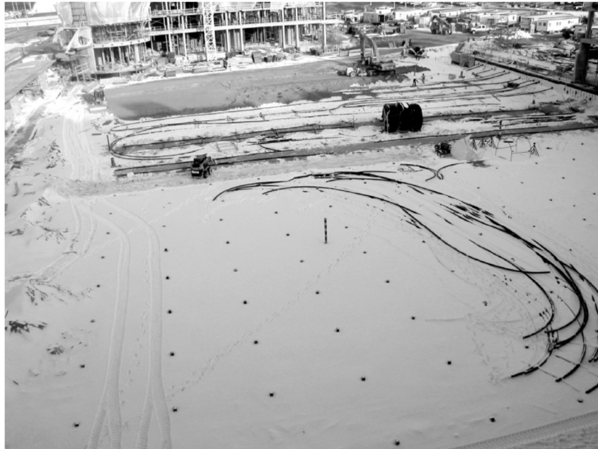
Figure 4-14: A site view during construction of the BTES in Canada [23].
