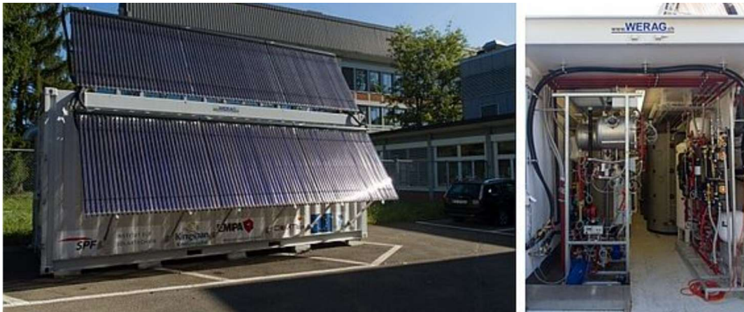
Figure 5-11: Pilot-scale storage plant combining long-term sorption storage and short-term sensible designed to cover yearly energy demand of a low-energy single family home [52].
